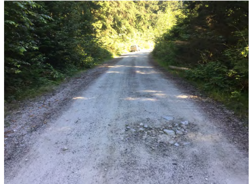
Right Approach Facing Away From Culvert
