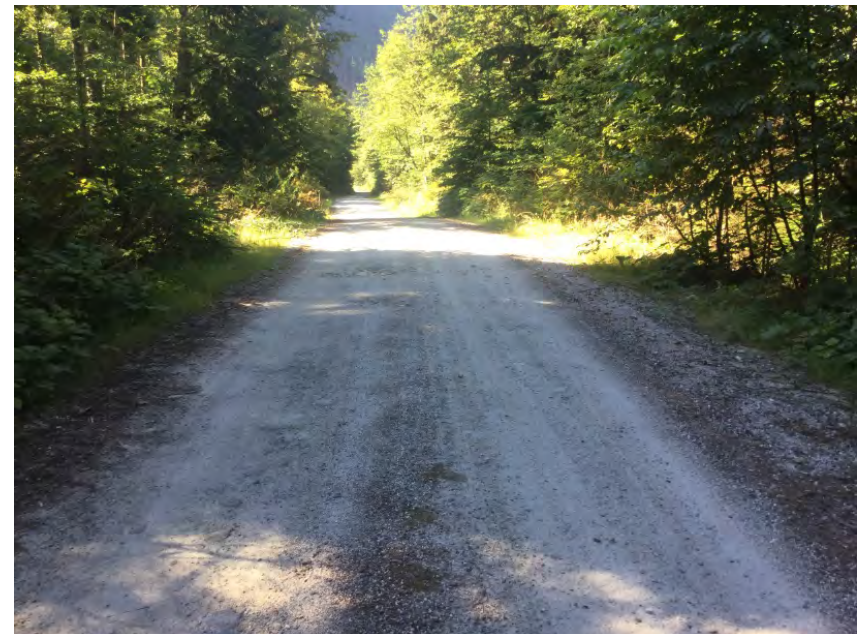
Right Approach Facing Culvert
