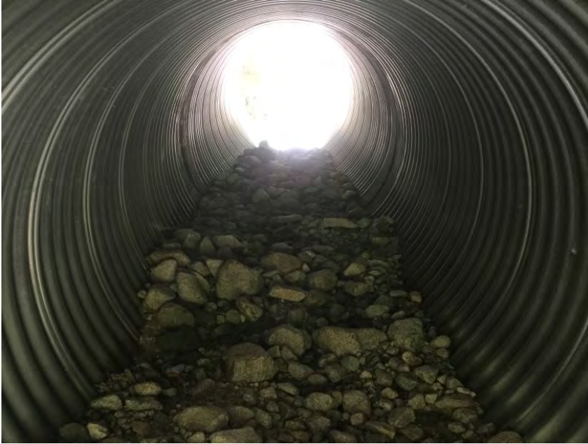
Barrel of Culvert 2
