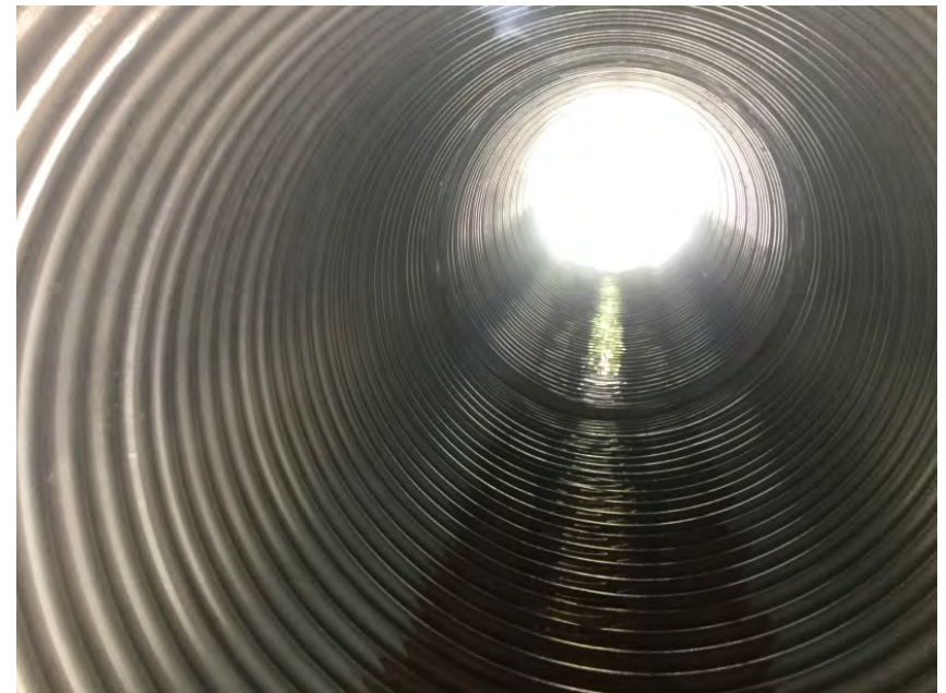
Barrel of Culvert 1
