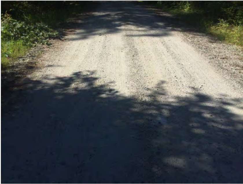
Roadway Over Culvert
