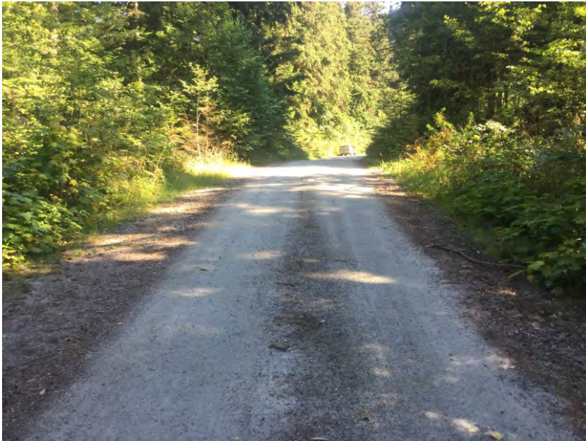
Left Approach Facing Culvert
